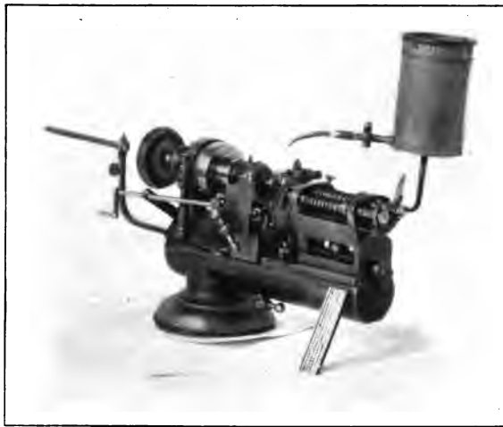
Fig. 36. Early Form of Screw Cutting Lathe.
