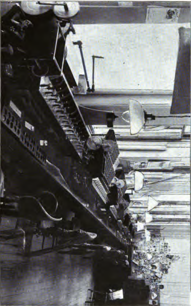
Fig. 60.—Balance and Hair Spring Vibrating Machines.
